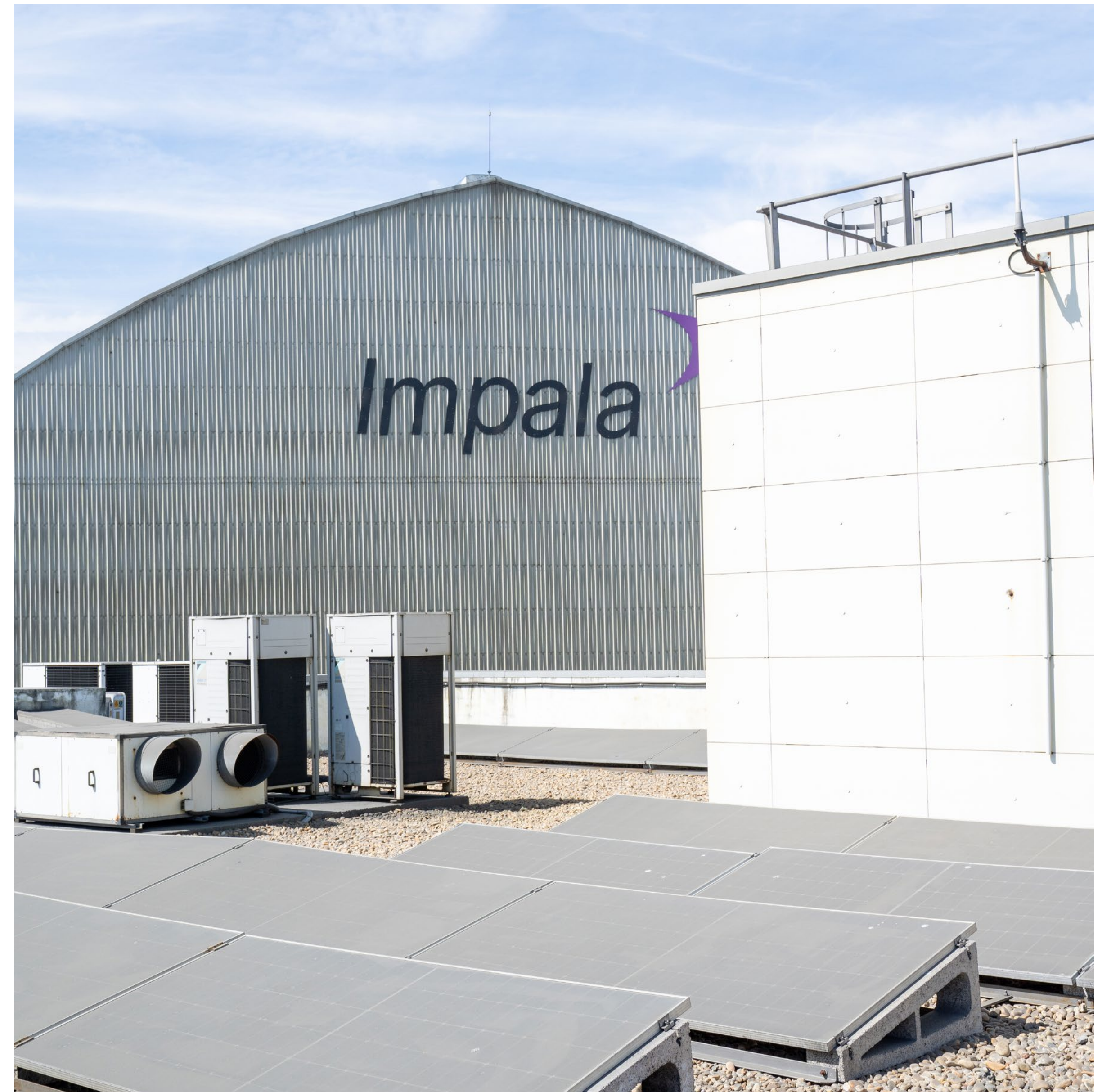
Impala Terminals Huelva, Spain
