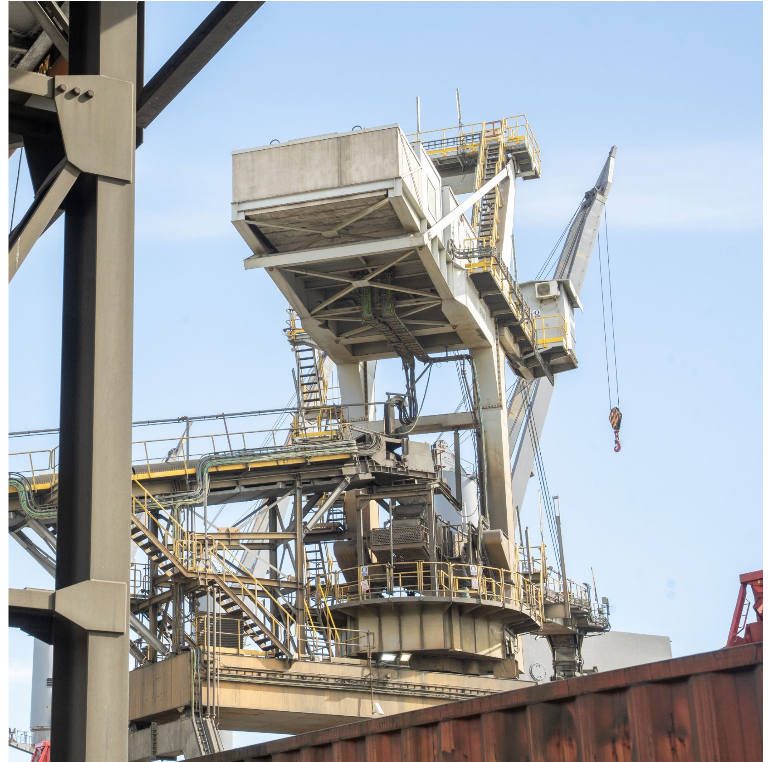
Impala Terminals Huelva, Spain
