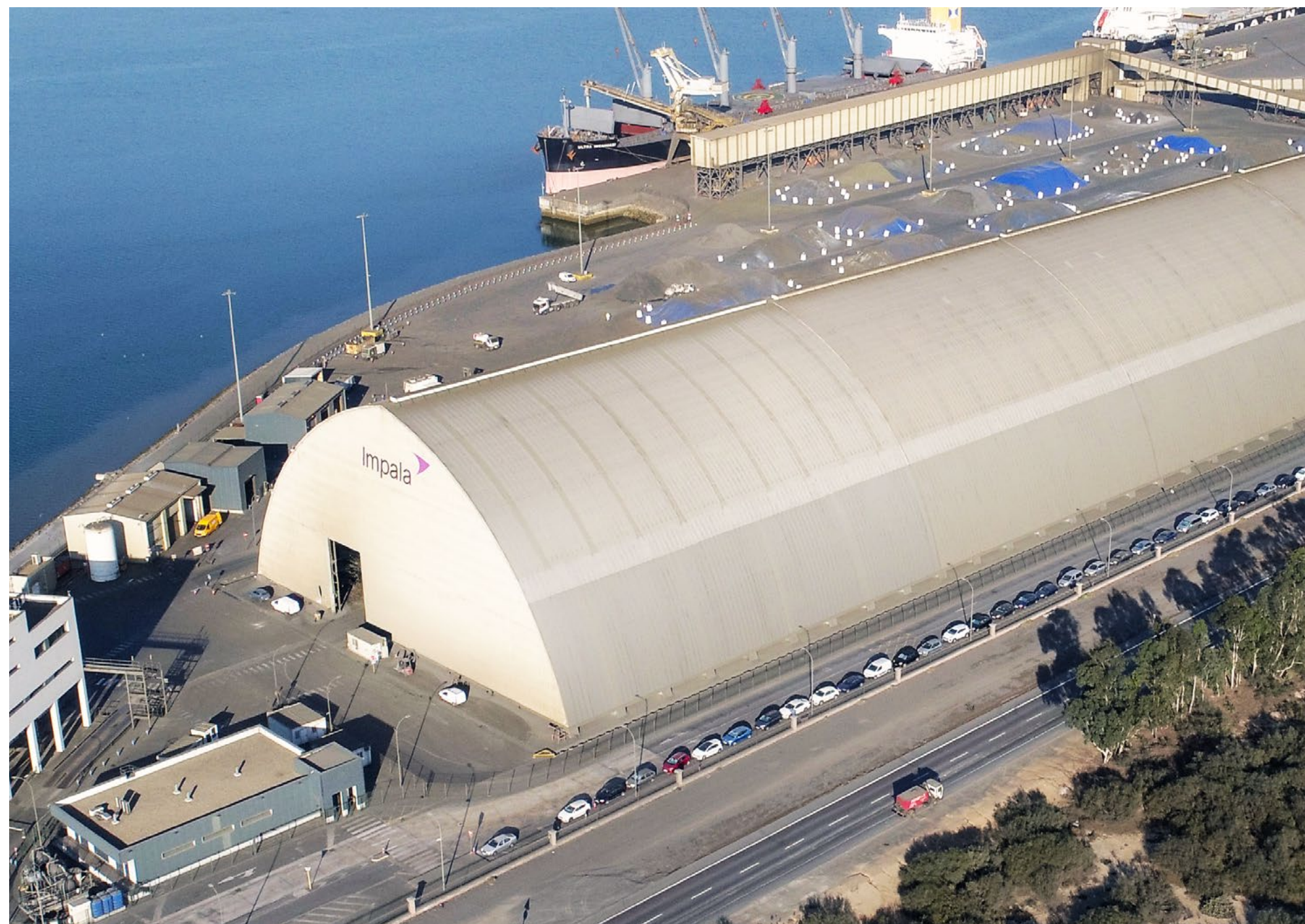
Impala Terminals Huelva, Spain
